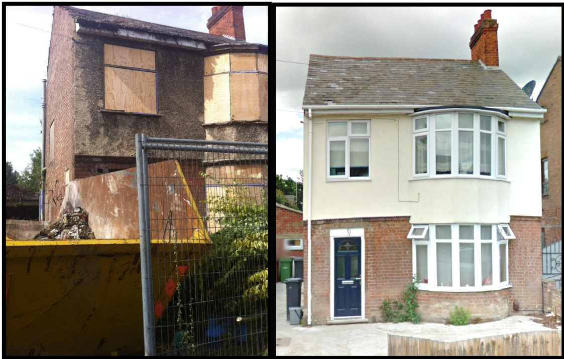
Fletton Avenue - Empty for 2 years and brought back into use through enforced sale and refurbished by the new owner
